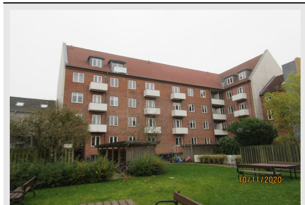
Altaner, facade mod baggård
